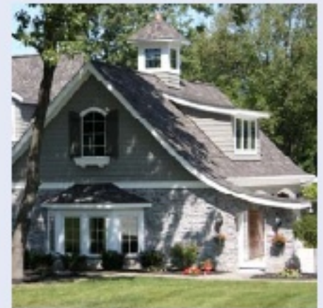
Partial Front Facade
